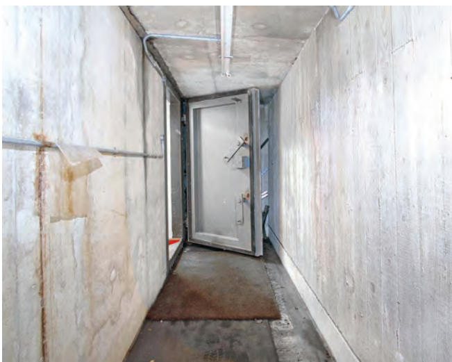
Looking out of the bunker from the dog-leg corridor After the airlock there are two routes into the bunker,
